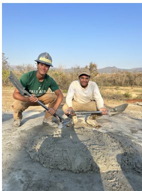
On-site cement mixing
