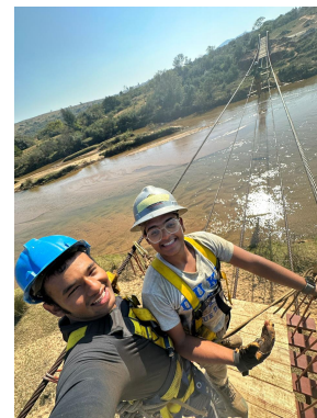
Installing the floor deck
