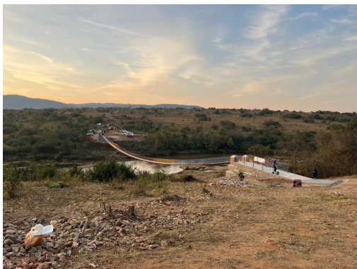
Completed 122 m bridge
